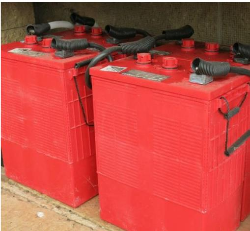
Deep cycle batteries should last more than ten years when properly maintained.
